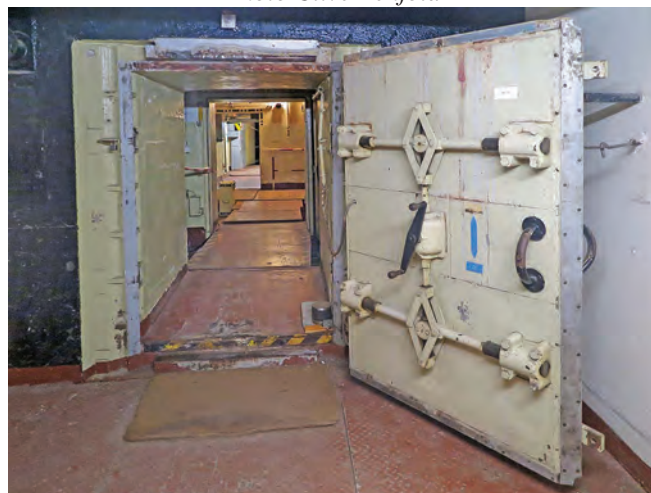
The blast door between the Harnekop bunker and the access tunnel. Photo Clive Penfold
